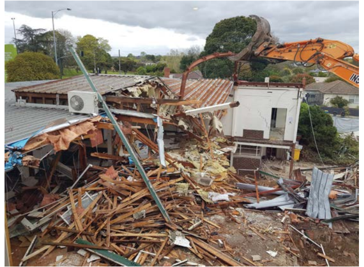
Demolition well under way!
